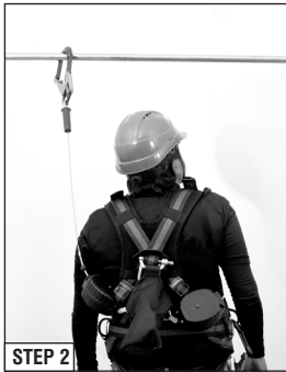
STEP 2 Work on single lanyard Park the unused, the second leg on to the harness's lanyard keeper. So that it does not gets entangled while working.
