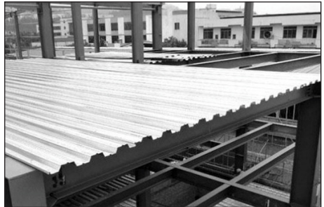
Steel deck and metal roofing
