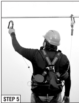
STEP 5 Completing Lateral Movement Now for further lateral movement along the line, disconnect the one leg from the first anchorage point and connect it to the successive anchorage point.
